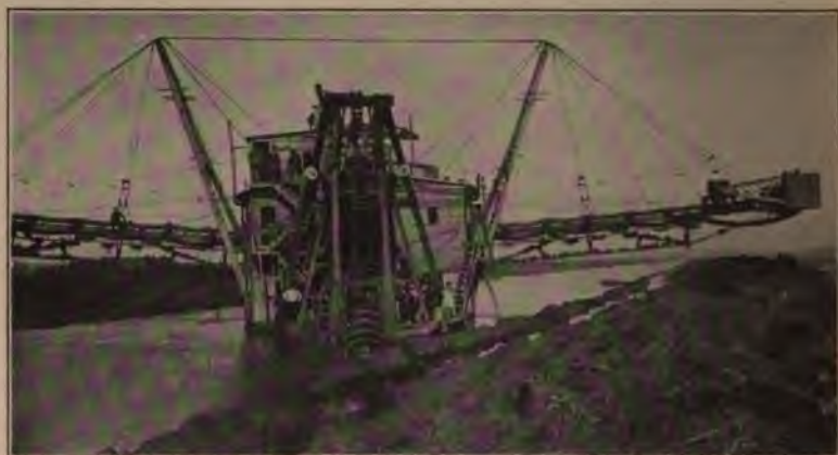
Elevator Dredge Excavating Large Drainage Ditch.
